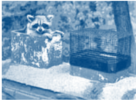
Raccoon coming out of a non-capped chimney. The other chimney has a wire-mesh cap to prevent animals from getting inside.
